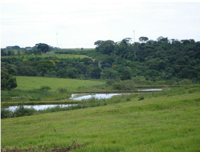
Figure 4. Present view of the dams.
